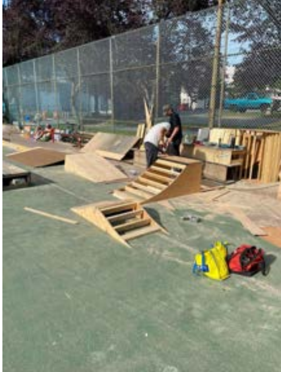
CONSTRUCTION OF OBSTACLES 1
